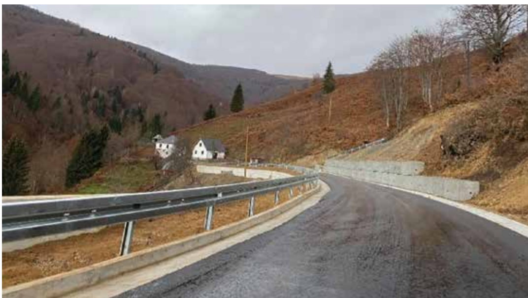
Supervision on the rehabilitation of the landslide “Gnjila Potok” on the road Mateševo – Andrijevića of a landslide approximately 140 m long, within which the reconstruction of the road structure was performed
